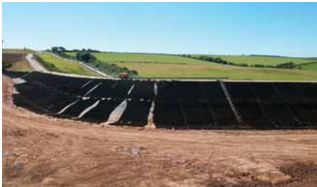
Geocell Panels positioned prior to fixing
