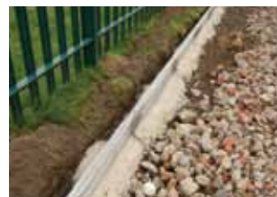
Edging kerbs installed
